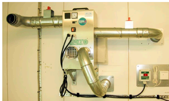
A DR-010B with DST humidistat EH4 controls moisture at a booster station
