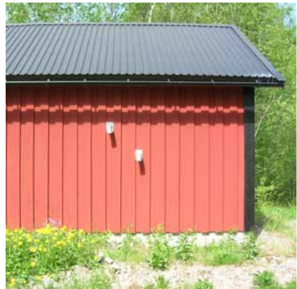
Wet air is fed out outside the booster station and regeneration air enters.
