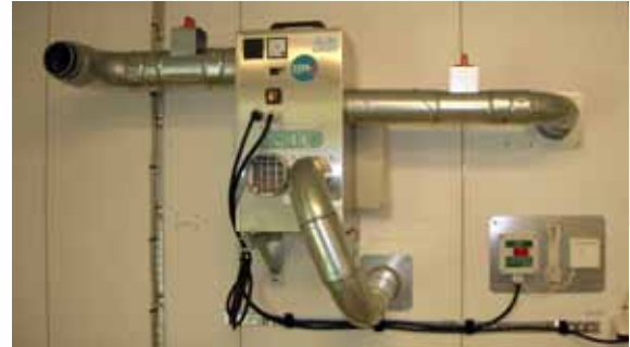
A DR-010B with DST humidistat EH-4 controls moisture at a booster station..
